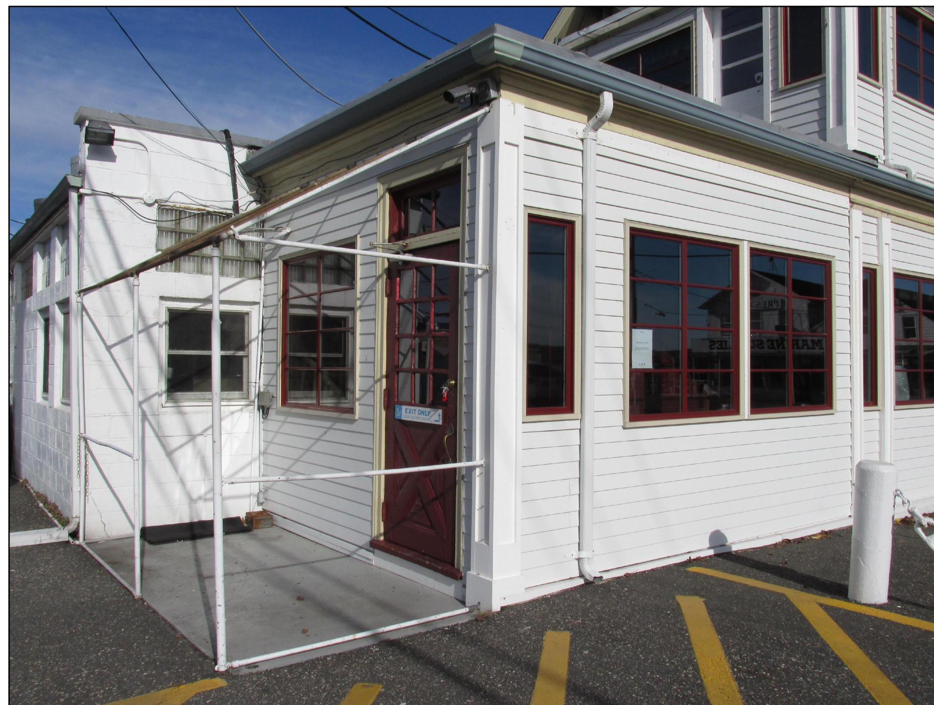
WEST ENTRY AWNING
