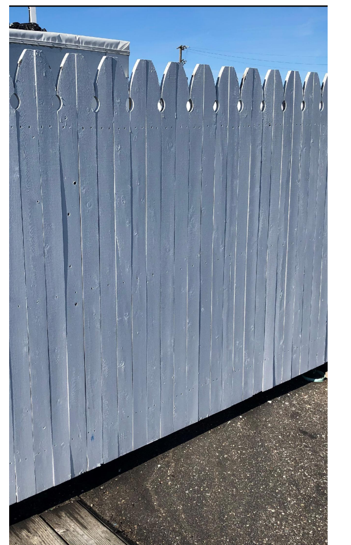
PROPOSED FENCE AT WALK-IN COOLERS TO MATCH FENCE AT CRABBY JERRY'S (SHOWN)
