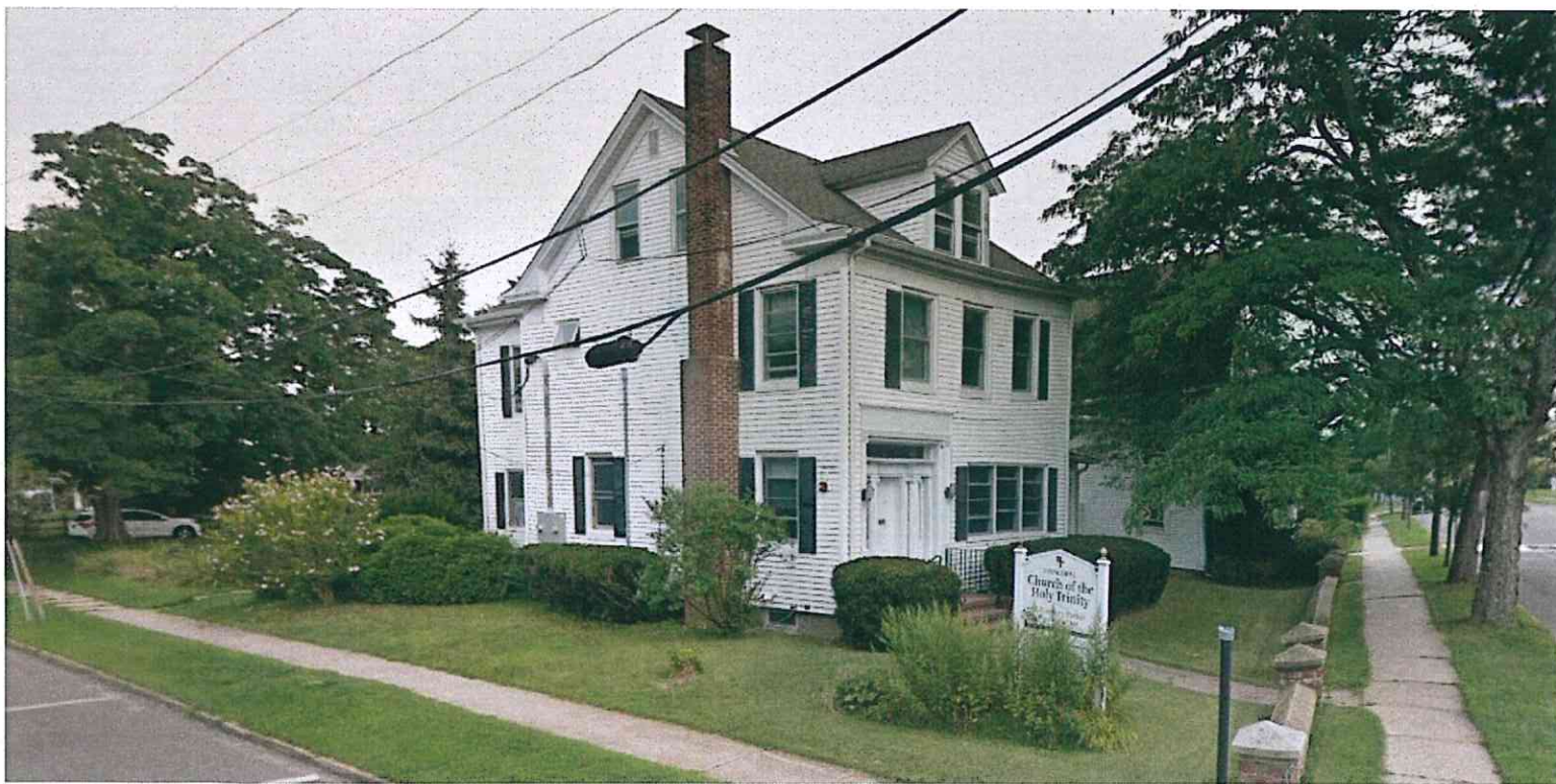
768 MAIN STREET (OPPOSITE PROPERTY)
