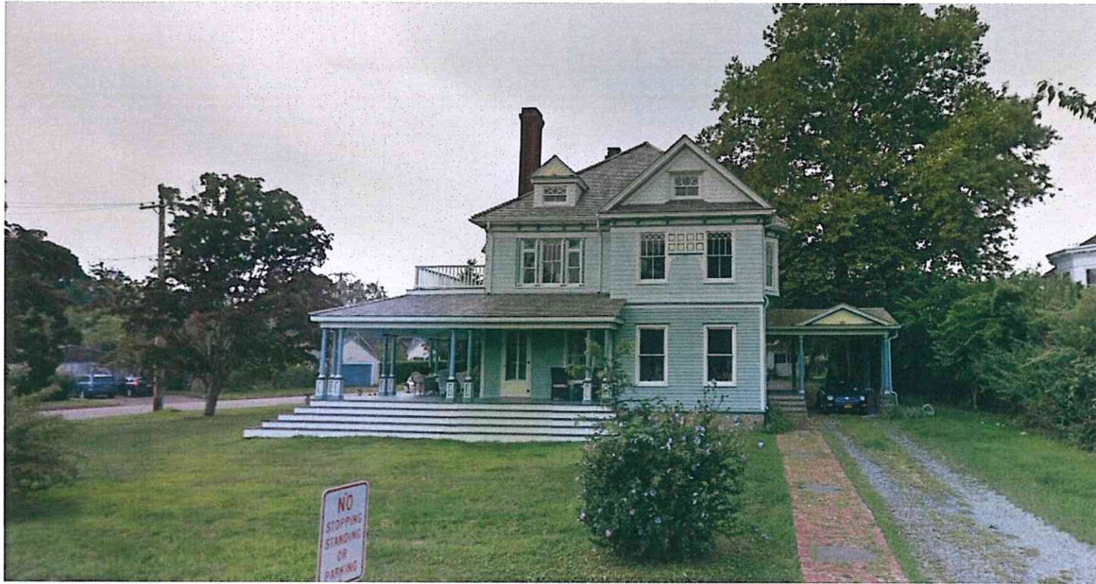
807 MAIN STREET (ADJACENT PROPERTY, SOUTH SIDE)
