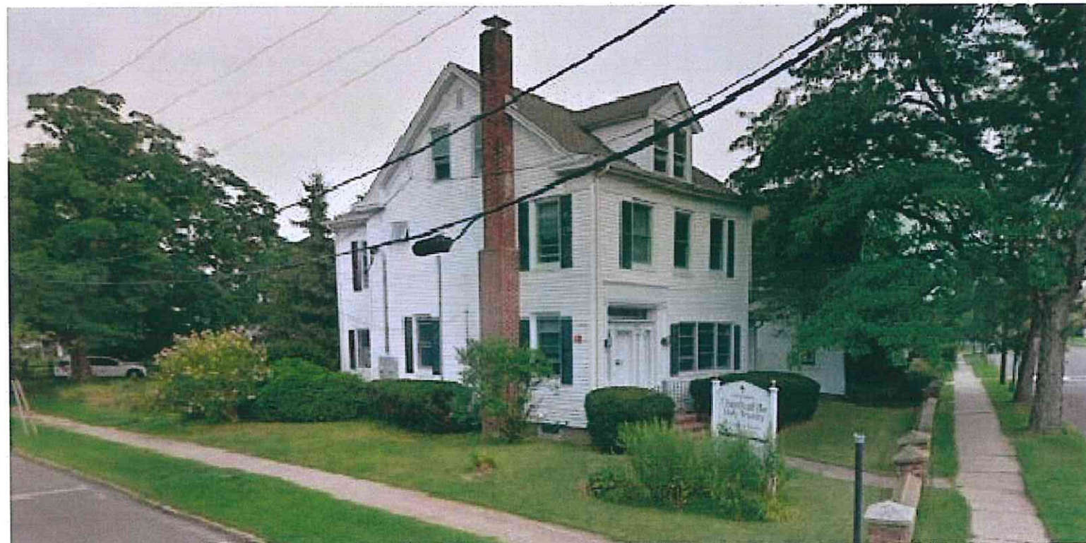
768 MAIN STREET (OPPOSITE PROPERTY)
