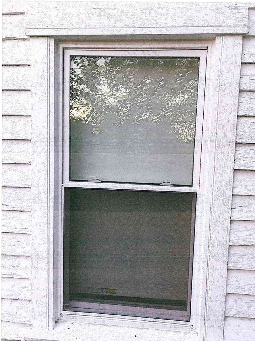
EXISTING WINDOW PREVIOUSLY INSTALLED ON EXISTING HOUSE
