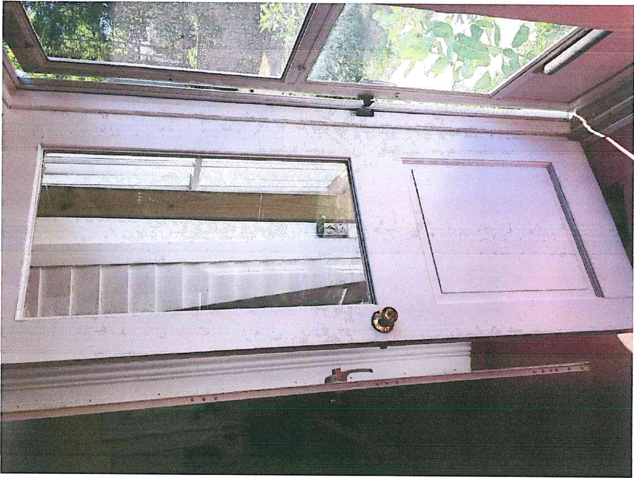
EXISTING WOOD EXTERIOR DOOR
