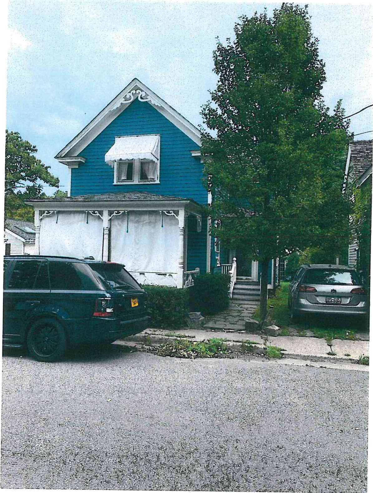
Current shed from street:
