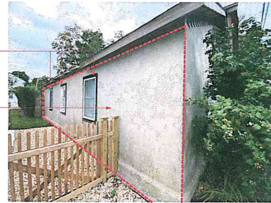
SIDE VIEW OF EXISTING MAIN HOUSE
