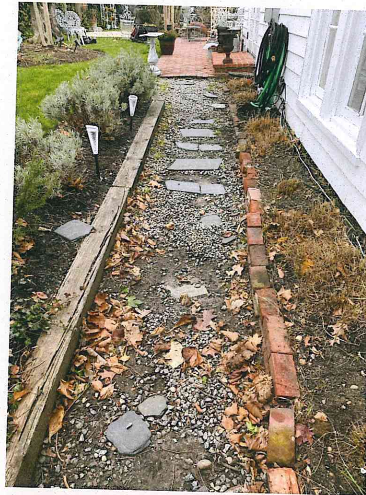
Existing path from trellis to garden area is uneven, and not designed for optimal drainage. Currently grade slopes toward building and may lead to water damage at foundation.
