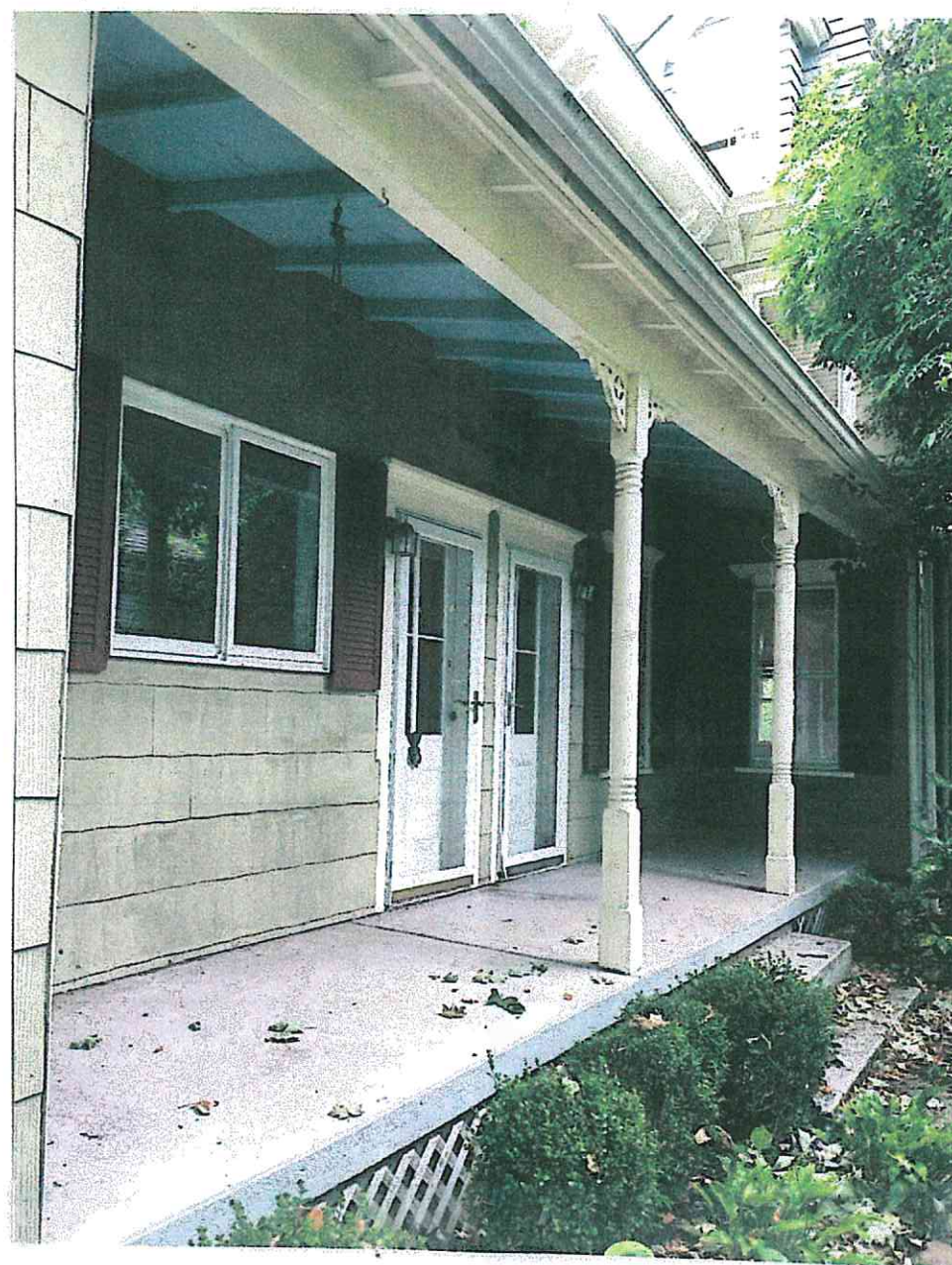
148 BAY AVE - SIDE PORCH - SOUTH
